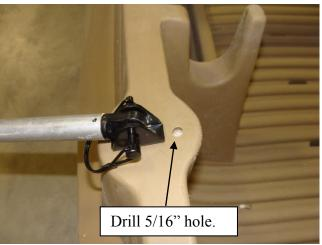
5. Insert brass insert, slotted end up, into the hole and tap in with a hammer to get it started. Make sure it is going in straight. Thread the insert into the hole with a flathead screwdriver. Install the ½ x 1 ½" fully threaded bolt into the insert and place the plastic cap on top of it. Note: This will adjust the height of the door frames.
